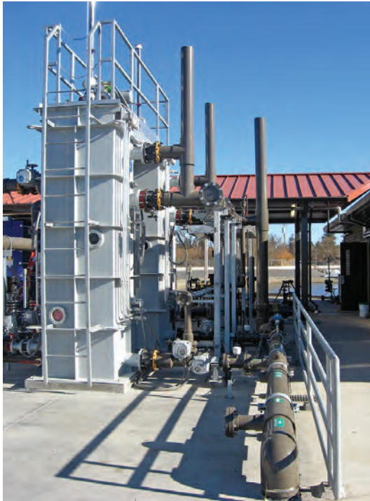
Fuzzy Filter simple depth filter technology (Schreiber) provides robust treatment with low energy and maintenance requirements.
